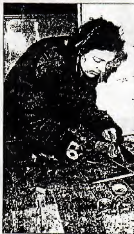
WORK UNDER WAY: Student Pippa helps with the renovations.
